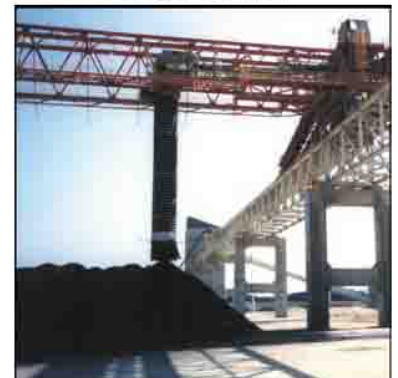
Stockpiling of coal with use of a tripper conveyor.
