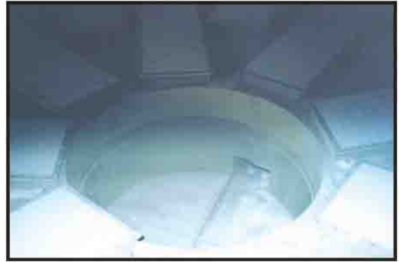
Aerated bin bottom silo discharge.
