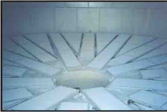
DCL's flat bottom silo aeration configuration, typical for all three silos.
